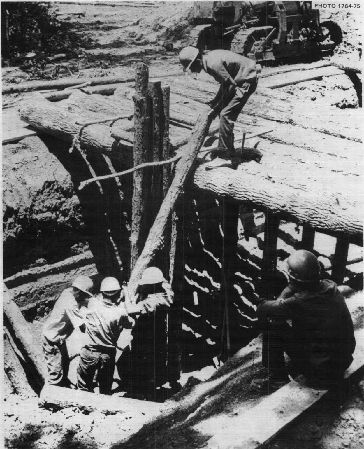
Fig. 7.2. Starting to erect one side of an entryway, after all of the 22-ft roofing logs had been positioned. A vertical entryway was placed at each end of the 12 × 42 ft shelter room.
